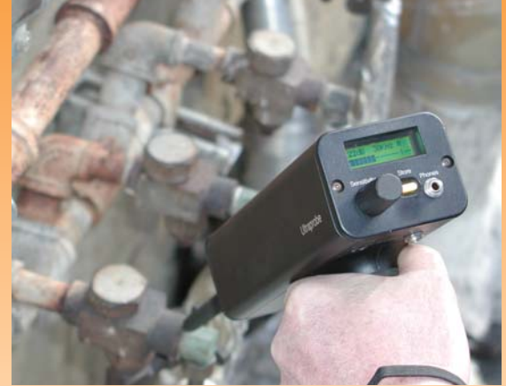
Inspect steam traps
